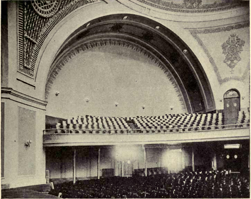
FIG. 4. PHOTOGRAPH SHOWING THE SIDE WALL OF FIG. 2 WHEN COMPLETED. A REP OF SUITABLE COLOR WAS STRETCHED OVER THE ENTIRE SURFACE AND DECORATED. IT WAS NECESSARY FOR THE FREE PASSAGE OF THE SOUND THAT THE MATERIAL USED IN DECORATING SHOULD NOT CLOSE THE PORES OF THE REP
